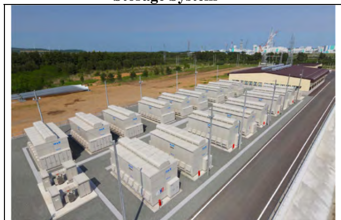
Figure 16-2. 34 MW Sodium-Sulfur Battery Storage System 627
