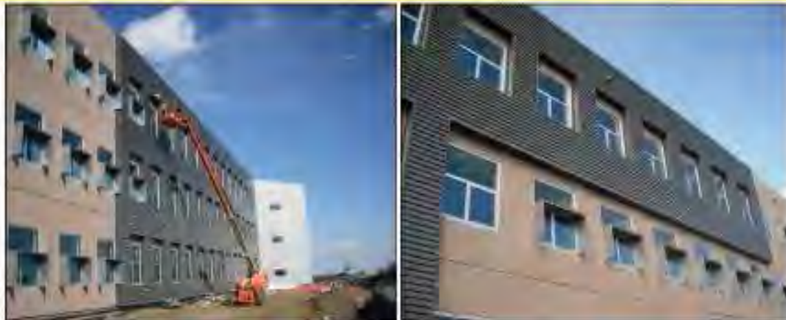
NREL's LEED Platinum Plus Research Support Facility showcasing innovative green technologies such as the SolarWall® solar air heating system (above, the two south facing charcoal SolarWall® systems)
