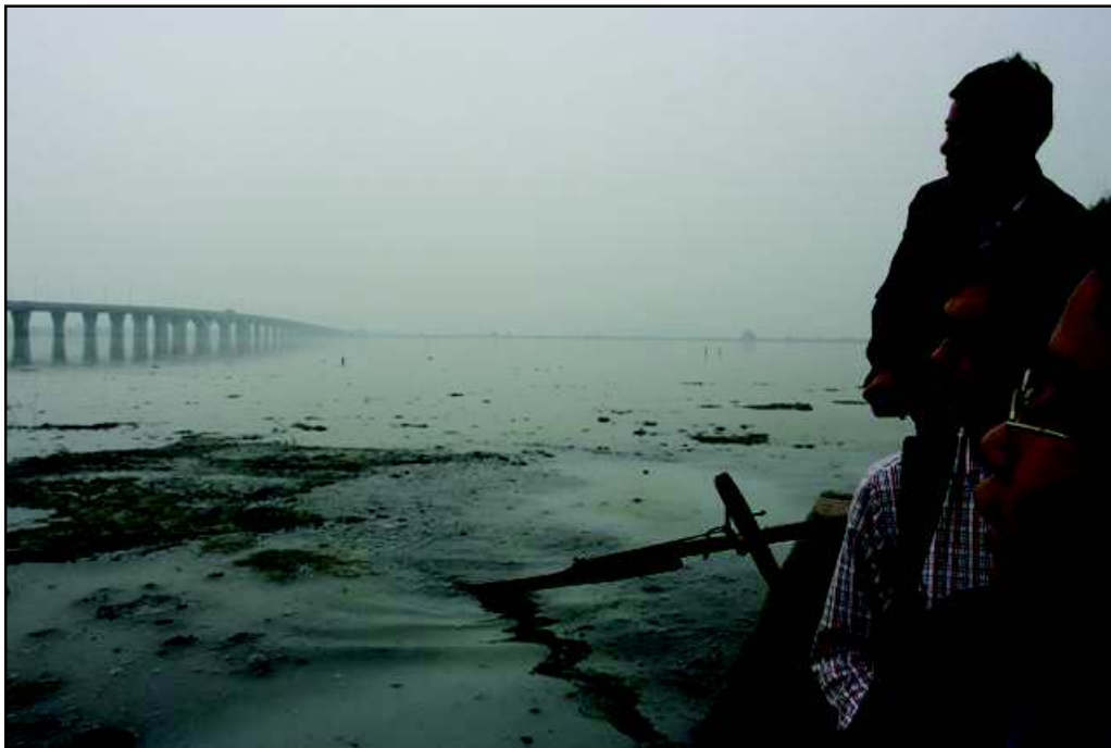
Figure 5: On-site Investigation, Photo: Ma Jun
