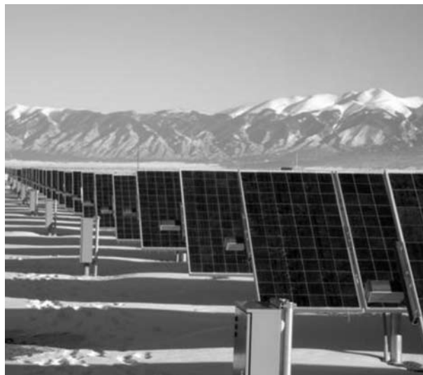
One-axis tracking photovoltaic panels at the SunEdison photovoltaic power plant near Alamosa, Colorado. Source: NREL.
