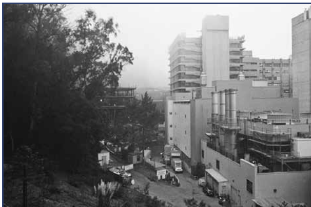
Combined heat and power unit at UC San Francisco. Photo by Susan Merrell/UCSF.
